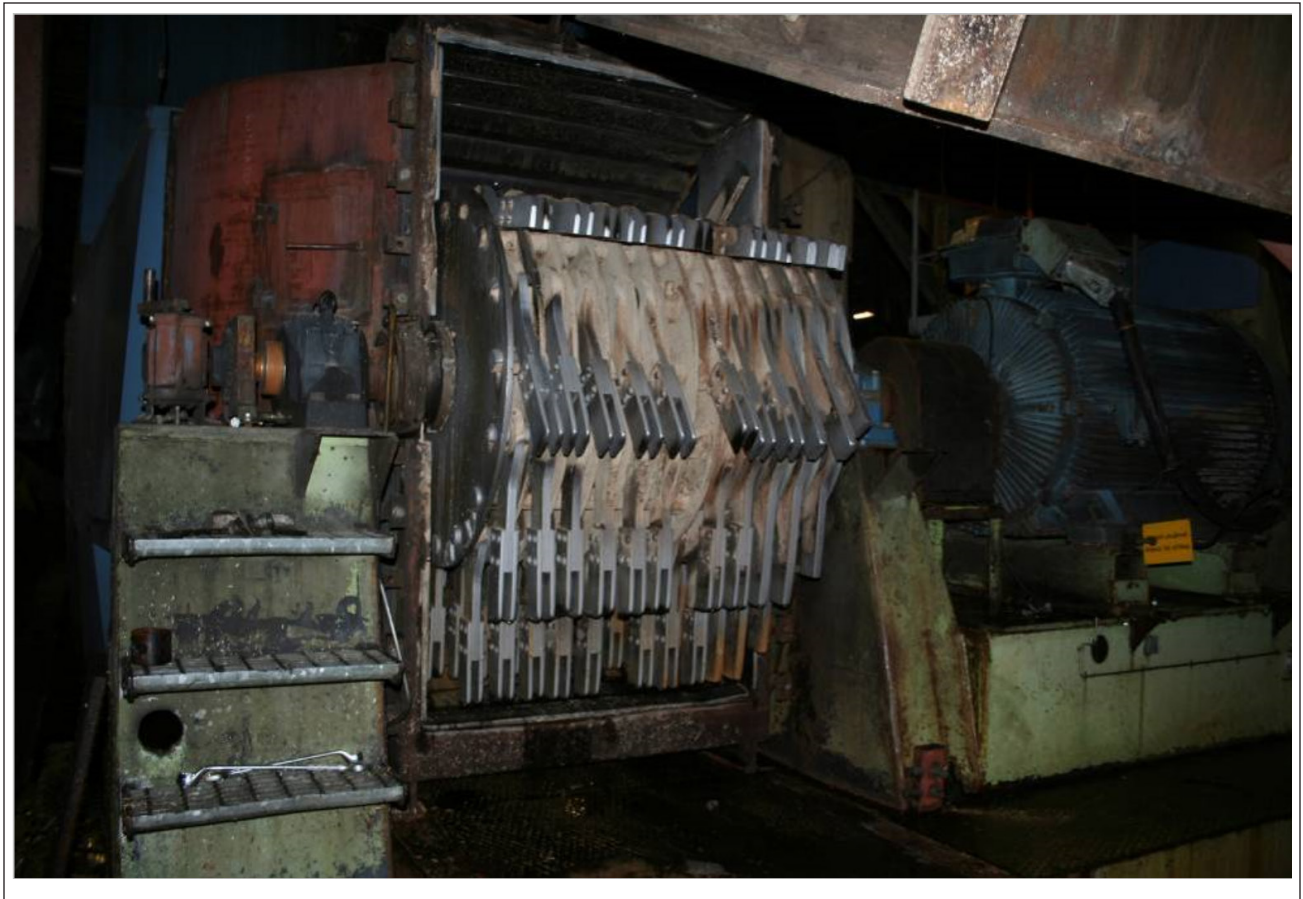
6. Hammer mill opened for inspection.
